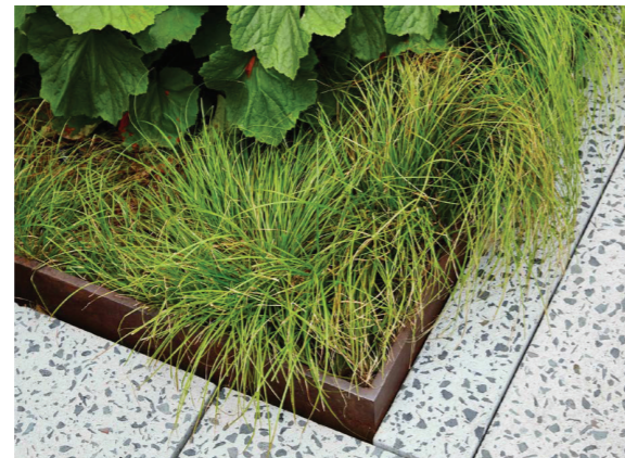
Figure 60: Cor-ten steel planter edge
