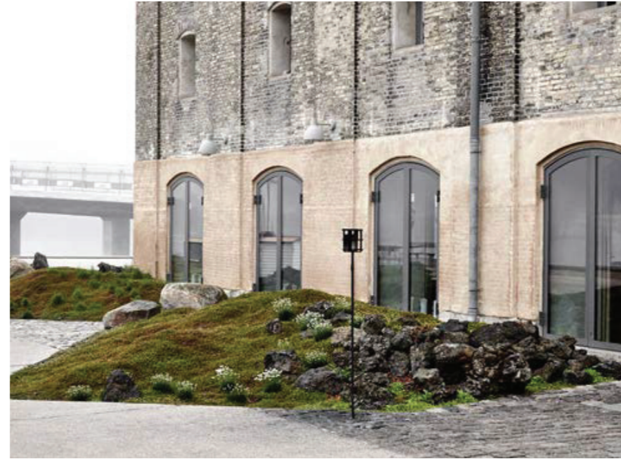
Figure 70: Soil mounding and rocks to screen private terraces in salvaged paving and exposed aggregate concrete
