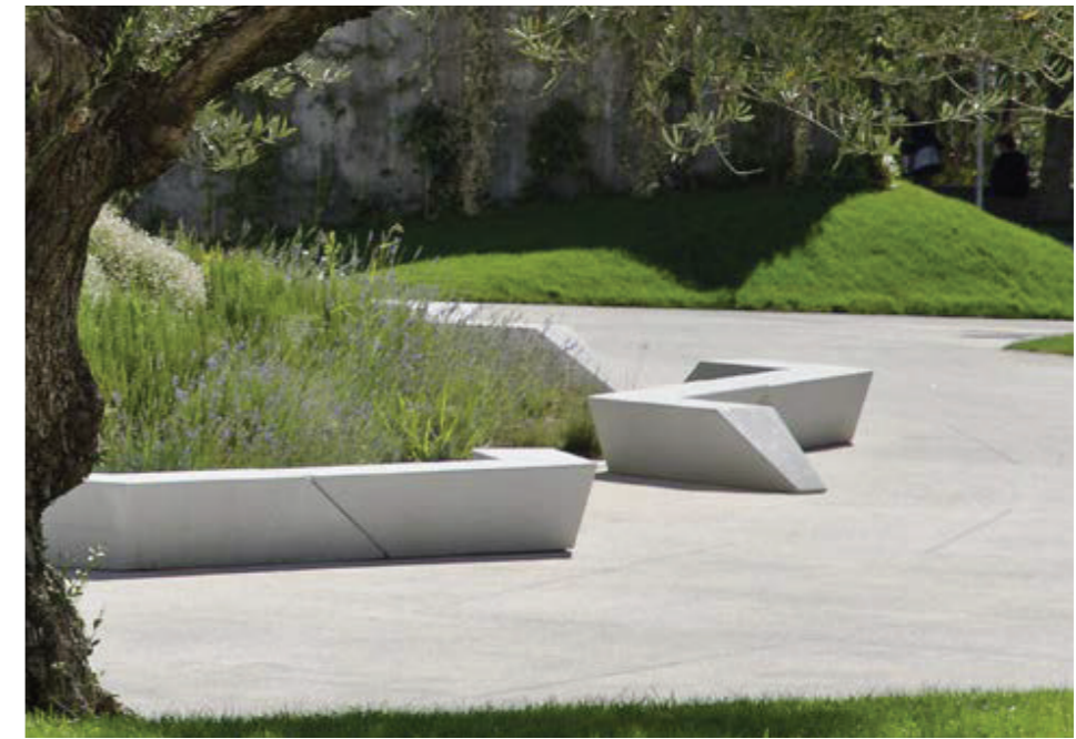
Figure 71: Precast concrete elements for soil mounding & seating
