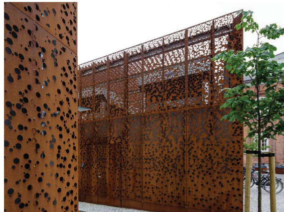
Figure 58: Cor-ten steel laser cut panels for screening or railing
