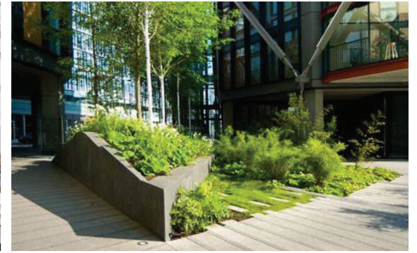
Figure 63: Raised concrete edge for deeper planting
